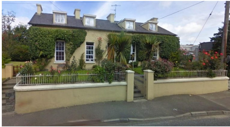
Plate 13-37: Recorded street house Killygordon, Reg. 40839004 (image Google Street, September 2009).
