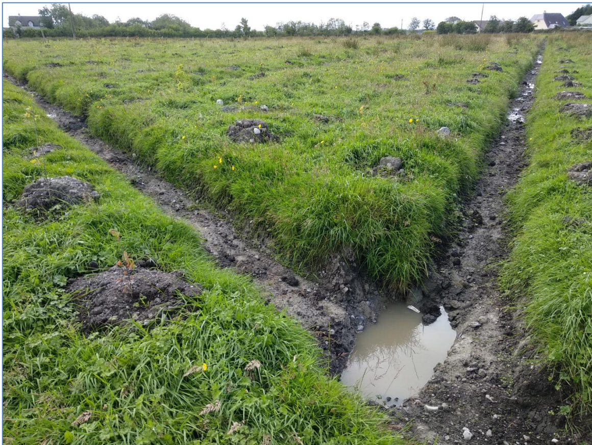
Plate 13-26: Recently planted saplings and associated drainage within re-planting Site 3 (from N).
