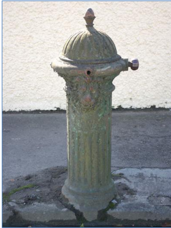
Plate 13-34: Close up of water hydrant, Reg. 40838038 (from www.buildingsofireland.ie ).
