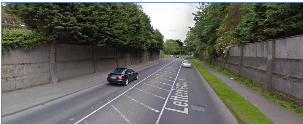
Plate 13-39: View of NW limits of Node 8. Note high mass-concrete walls on both sides (image from Google Street July, 2011).
