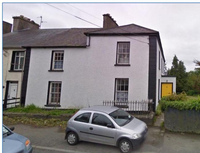
Plate 13-36: Tara House image (Google Street, 209-2011). Note majority of railings removed.
